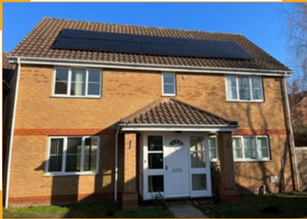
A house at the Mildenhall development, kitted out with solar panels.
